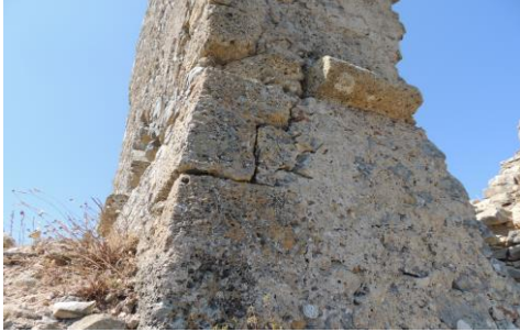
Fig. 3 – Tower of Capodomo: the corner stones and the cornice
