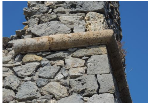
Fig. 10 – Tower of Calamoresca: dressed stone of the masonry made of dark grey dolomite and cornice made of Cavernous Limestone
