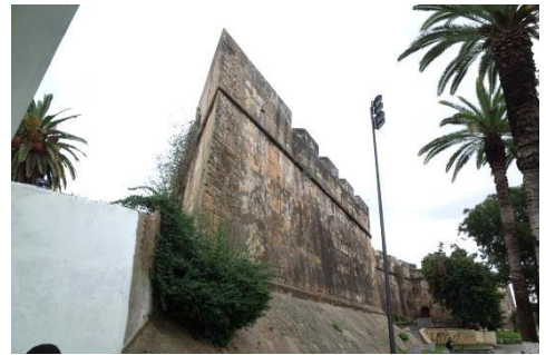
Figure 5- View of the southwestern bastion of the Hisn al-Nasr in Larache
