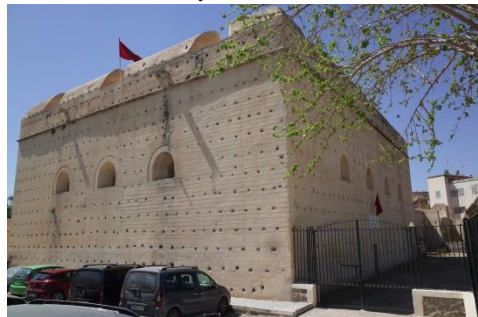
Figure 10- View of the bastion of Sheij Ahmad at Fes al-Jedid
