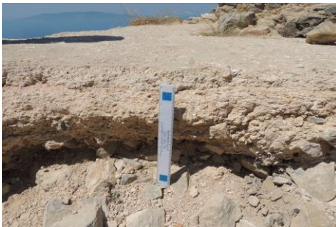
Fig. 4 – Tower of Capodomo: the two layers mortar flooring
