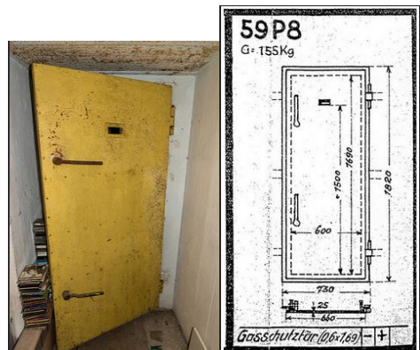
Fig. 11- Gas proof door type 59P8 with its original “Afrika Corps” sand yellow painting.
