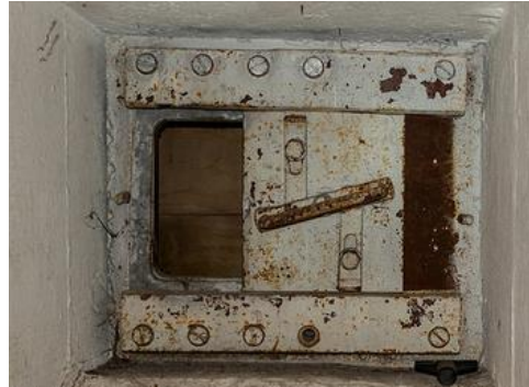
Fig. 14- Loop hole with locking system at double tenons joint and velvet.
