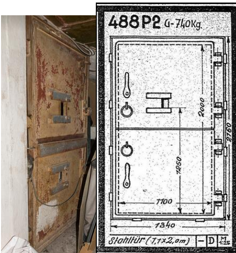
Fig. 13- Armoured door type 488P2 with double loopholes. The original paint is present: Antirust red primer layer and original "Afrika Corps" sand yellow painting layer. The isolating velvet is still in place on the edges.
