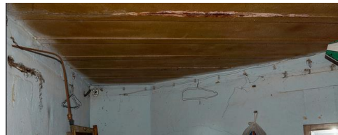
Fig. 16- Ceiling with metallic bars and original "Afrika Corps" sand yellow painting.
