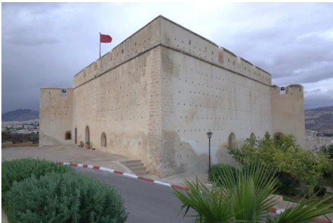
Figure 9- View of the southern side of the Burj South in Fes
